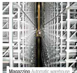
Magazzino Automatic warehouse
